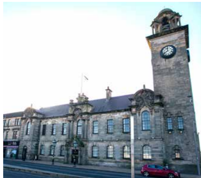
Completed improvement works at Clydebank Town Hall and increased exhibition space
