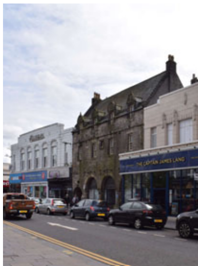
High Street. Glenclair House to centre
