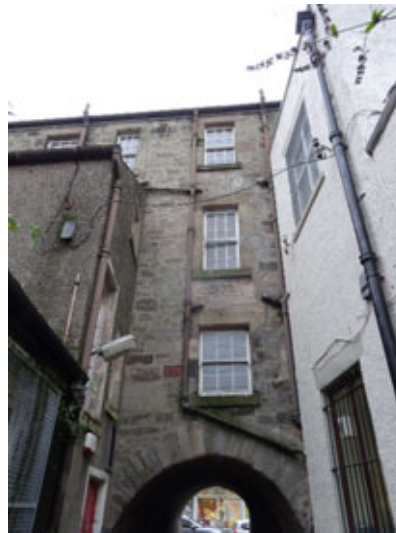
Rear elevation (east side above pend)
