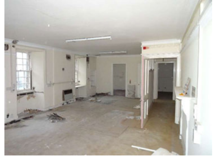
First floor. Principal room to High Street side (north)
