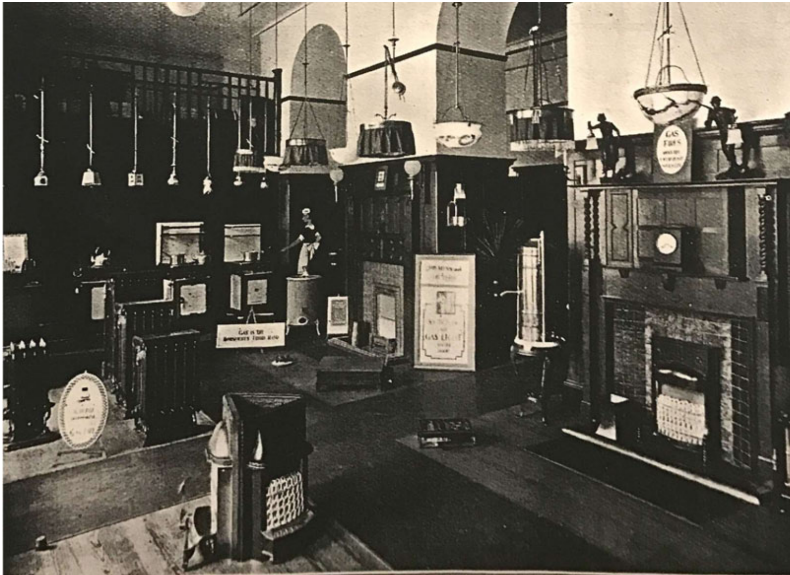
Figure 6: Internal view of the ground floor as display of domestic gas appliances. Gas Corporation c. 1925 West Dunbartonshire Council. Dumbarton Library Archive
