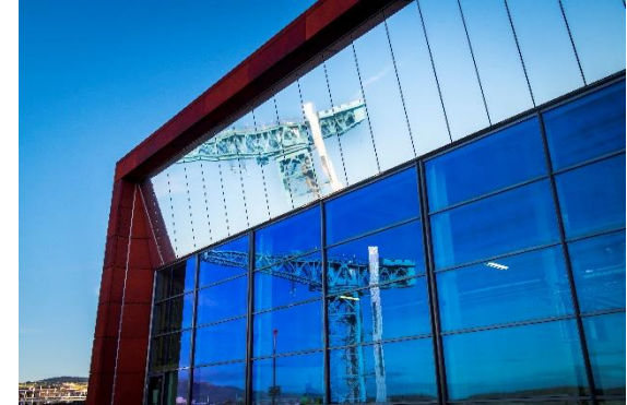
The Queens Quay Energy Centre. Clydebank supports an energy network for the whole Queens Quay site with network connections available for sites to the north of Glasgow Road. The iconic design of the building makes it landmark at the waterfront to complement the Titan Crane.
