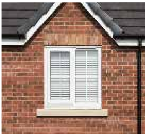
Not Preferred white PVC Windows or coloured UPVC windows with sightlines 10% greater than aluminium equivalent.
