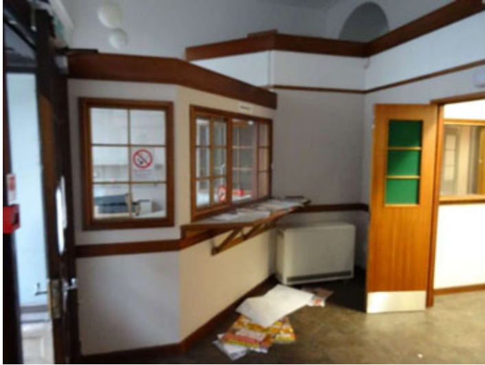
Ground floor (non-loading bearing partition sub-division)
