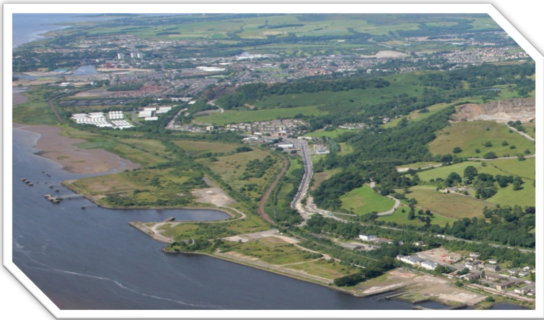
Figure 1-1 Exxon Site Aerial View
