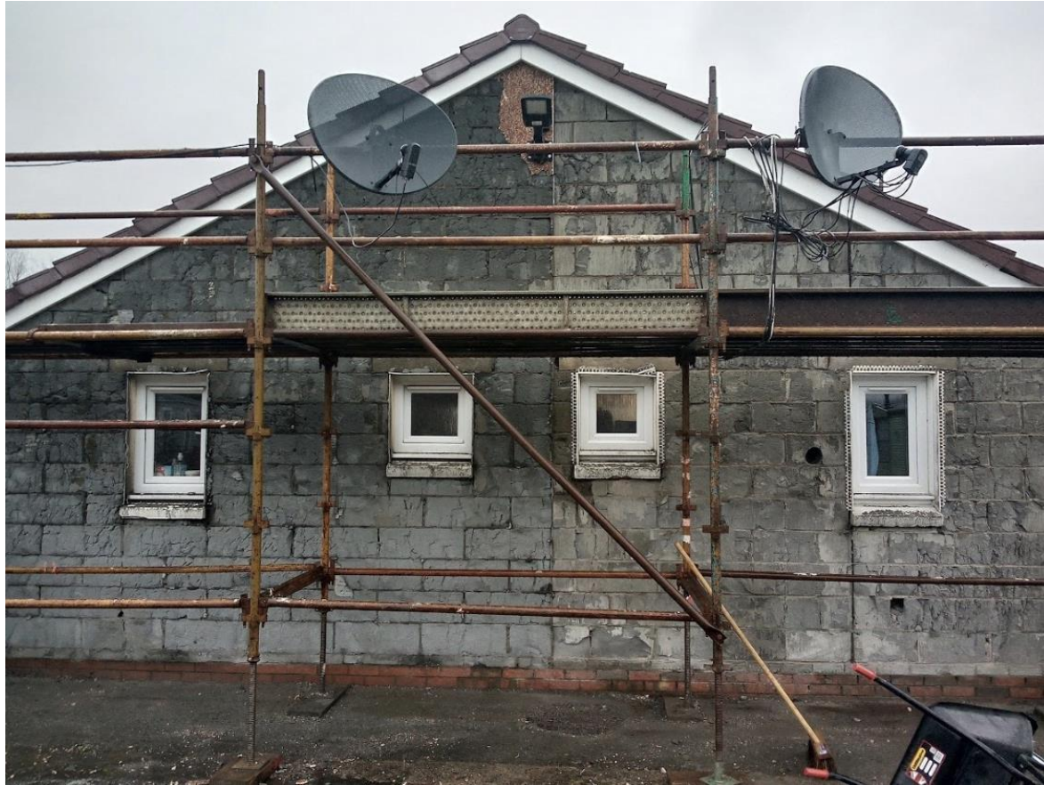
Picture showing a house stripped back to brick externally, new windows fitted and roofing works underway
